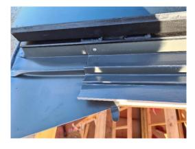
3. Fold tab of bottom flashing over edge of side flashing to hold in place.
