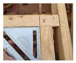
2. Install roof battens 5mm short of the frame opening size on all four sides. (Skylight is fixed into position on top of roof battens for both tiled and metal roofs)
